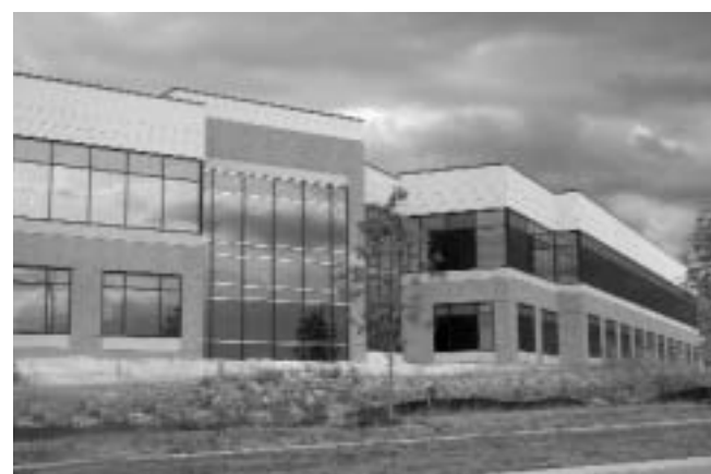
Two new buildings—which will house Terracon and a Garmin division (above, top) and Farmers (above)—will be complete before the end of the year.
